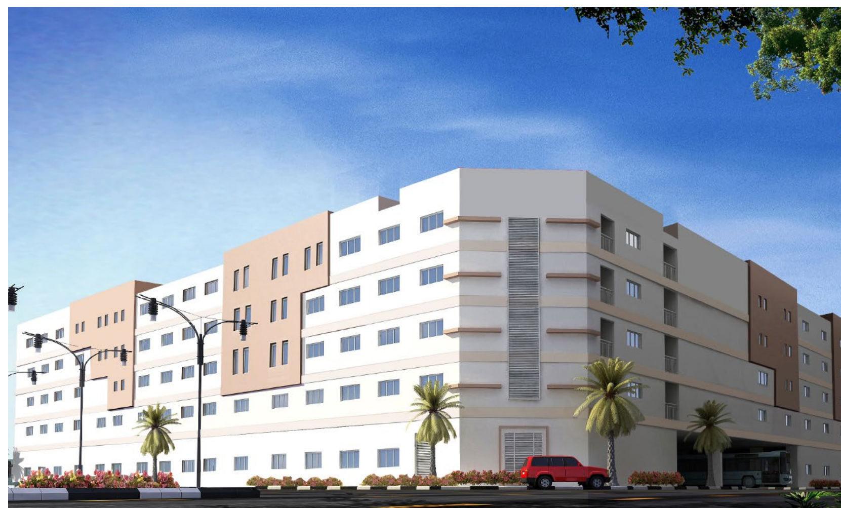
Labor Accomodation, Dubai-United Holdings
