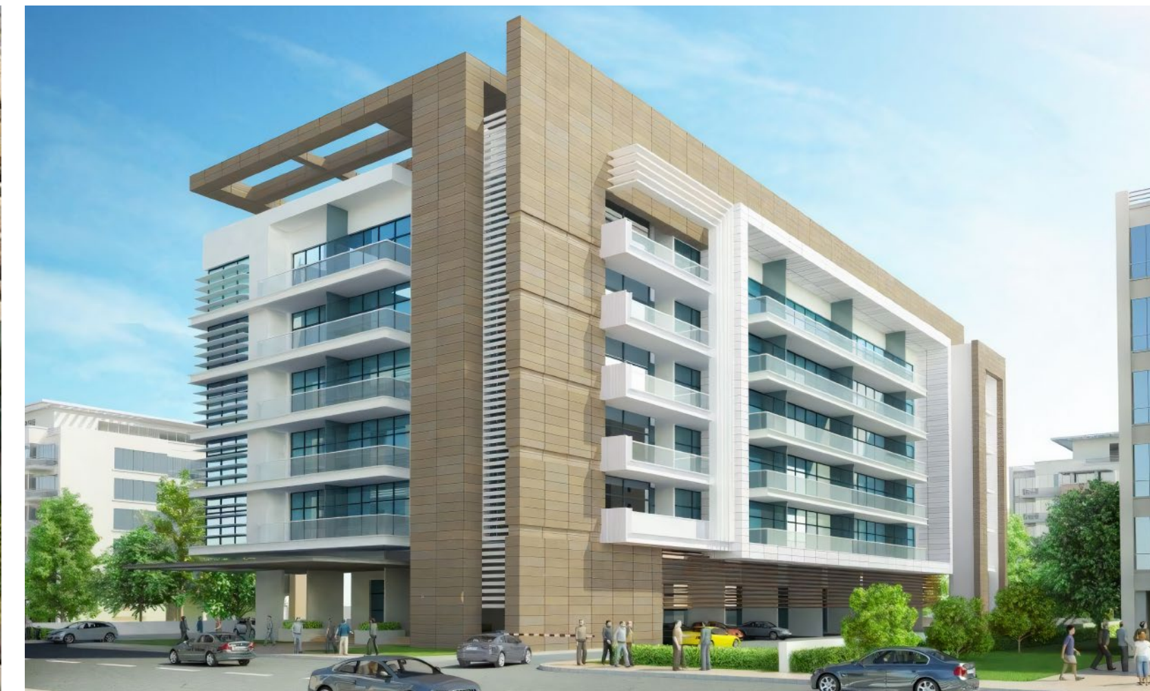
Residential building, Dubai Investments Park
